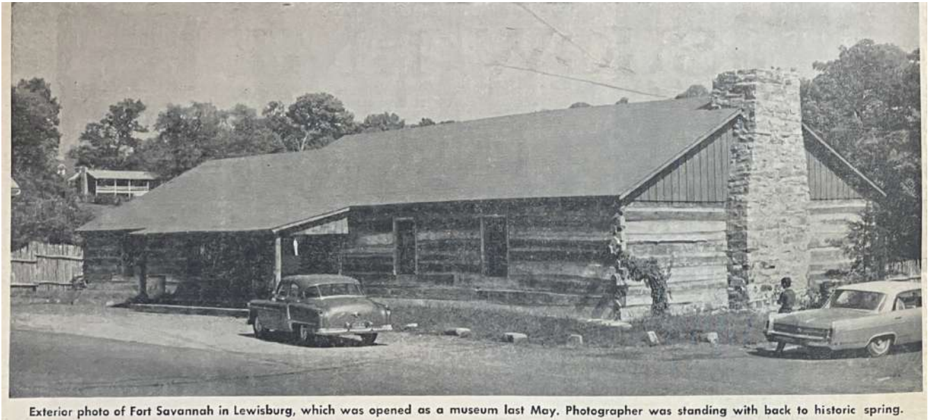
Exterior photo of Fort Savannah in Lewisburg, which was opened as a museum last May. Photographer was standing with back to historic spring.
